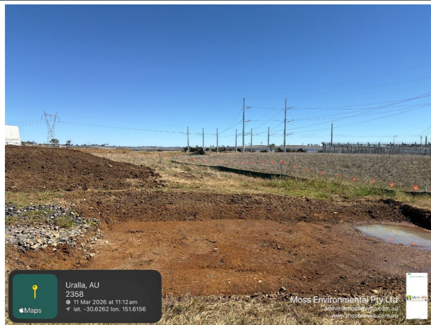
Photo 22 – Silt fence line around BESS
