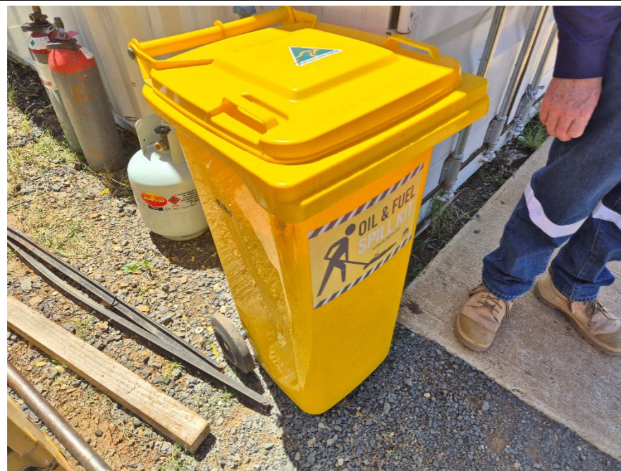
Photo 16 – Spill kit at the chemical storage area
