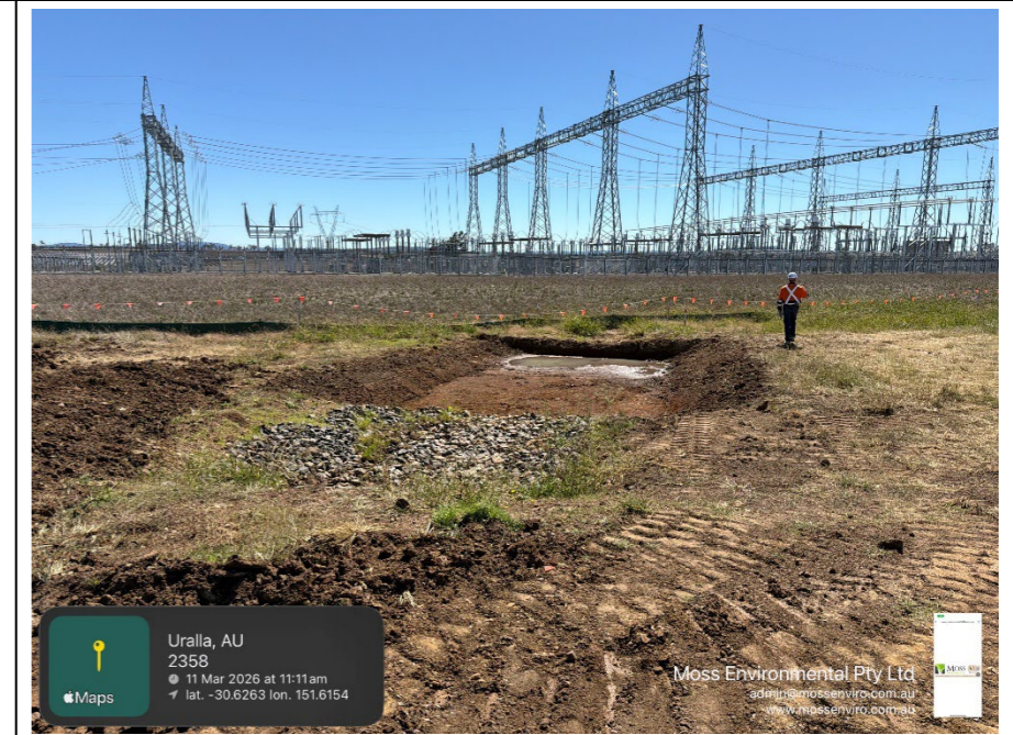
Photo 21 – Silt trap to the north of BESS
