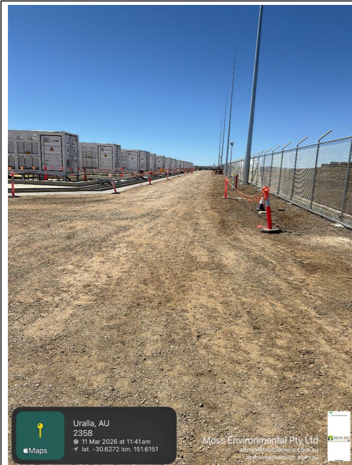
Photo 1 – All-weather roads are well maintained
