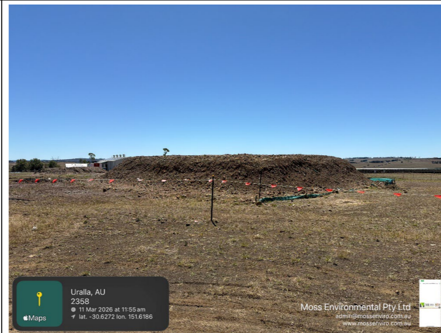
Photo 23 – Silt fence line damaged around the stockpile area
